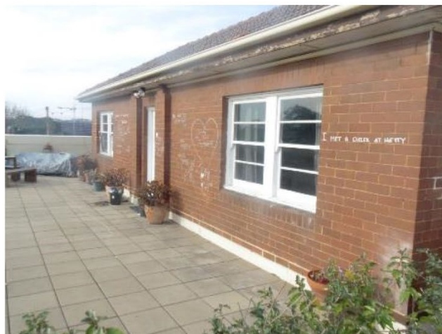
Roof terrace unit (ex. Caretakers residence)
