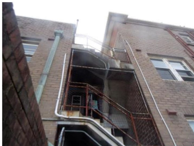
Rear service stairs
